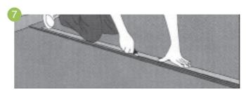
Position a straight edge along the middle of the overlap and cut through both pieces of carpet with a sharp knife and remove the surplus. Fold back the seam edges and apply adhesive onto the subfloor. Re-lay the carpet and roll with a 68kg flooring roller to ensure overall contact with the adhesive.
